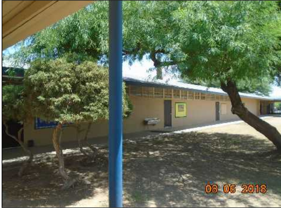
Picture 5 – South side exterior of Building 9 (RPA Building B – East).
