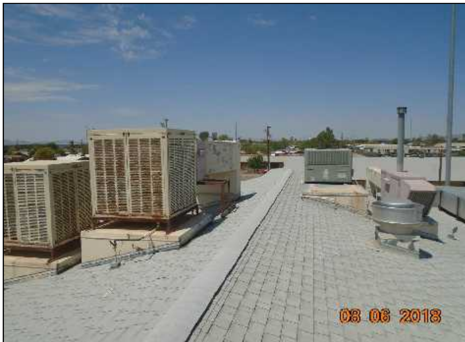
Picture 12 – Roof of Building 14 (RPA Building F).
