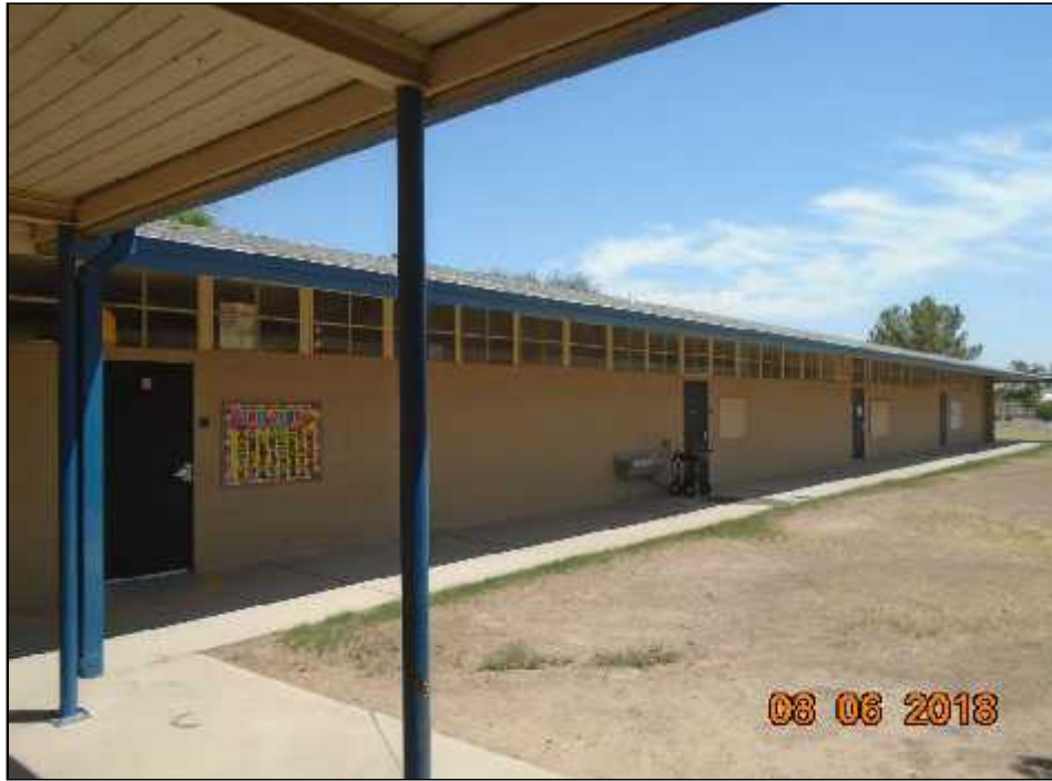
Picture 7 – South side exterior of Building 11 (RPA Building C – East).
