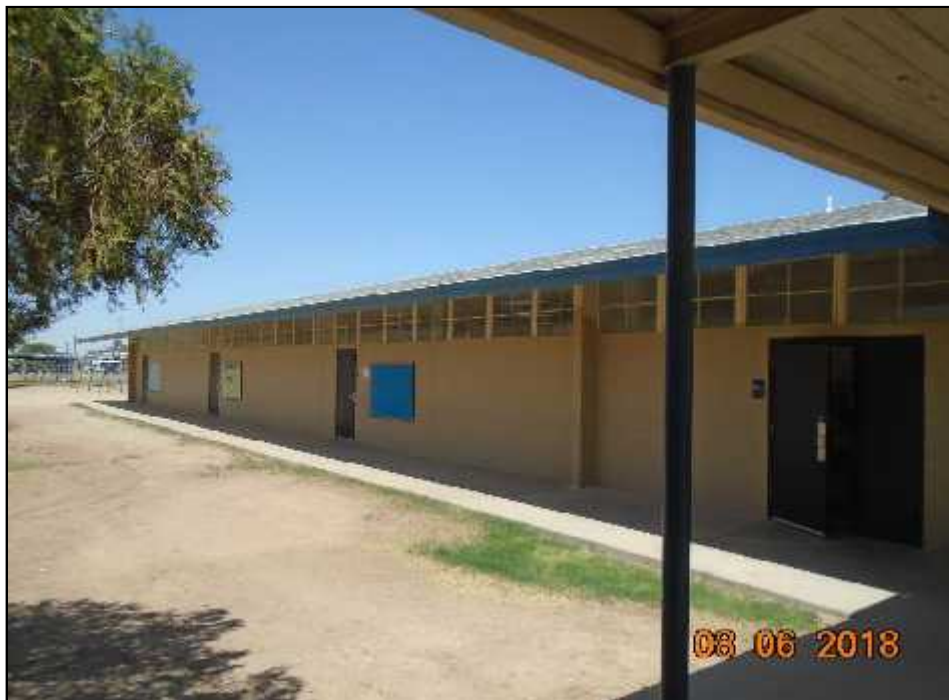
Picture 6 – South side exterior of Building 10 (RPA Building C – West).
