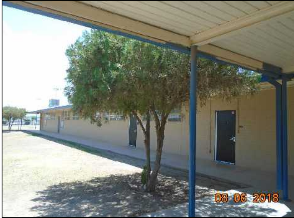
Picture 9 – North side exterior of Building 13 (RPA Building D – East).
