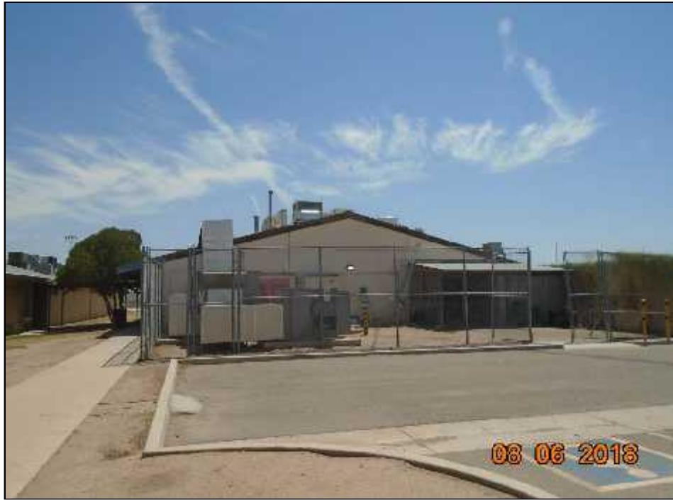
Picture 11 – West side exterior of Building 14 (RPA Building F).
