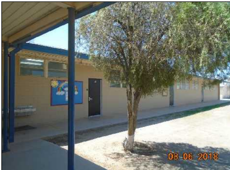
Picture 8 – North side exterior of Building 12 (RPA Building D – West).
