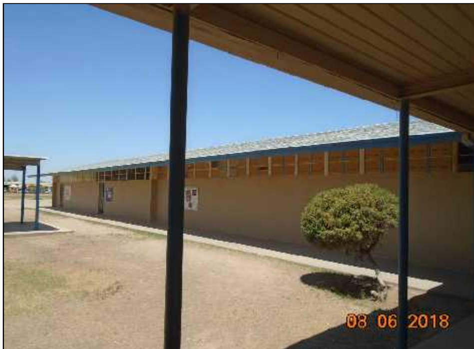
Picture 4 – South side exterior of Building 8 (RPA Building B – West).
