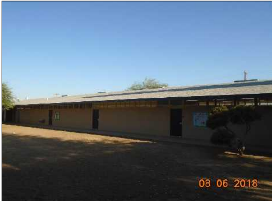
Picture 3 – South side exterior of Building 7 (RPA Building A – East).
