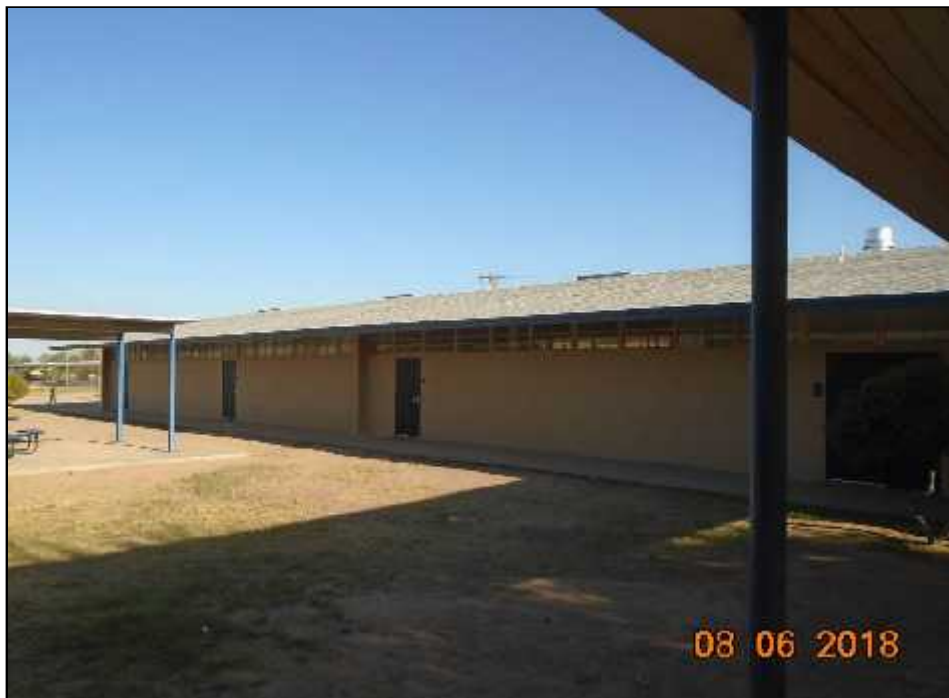
Picture 2 – South side exterior of Building 6 (RPA Building A - West).
