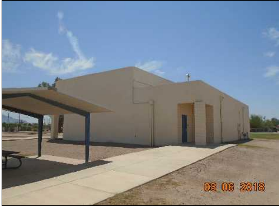
Picture 13 – South side exterior of Gymnasium (RPA Building G).
