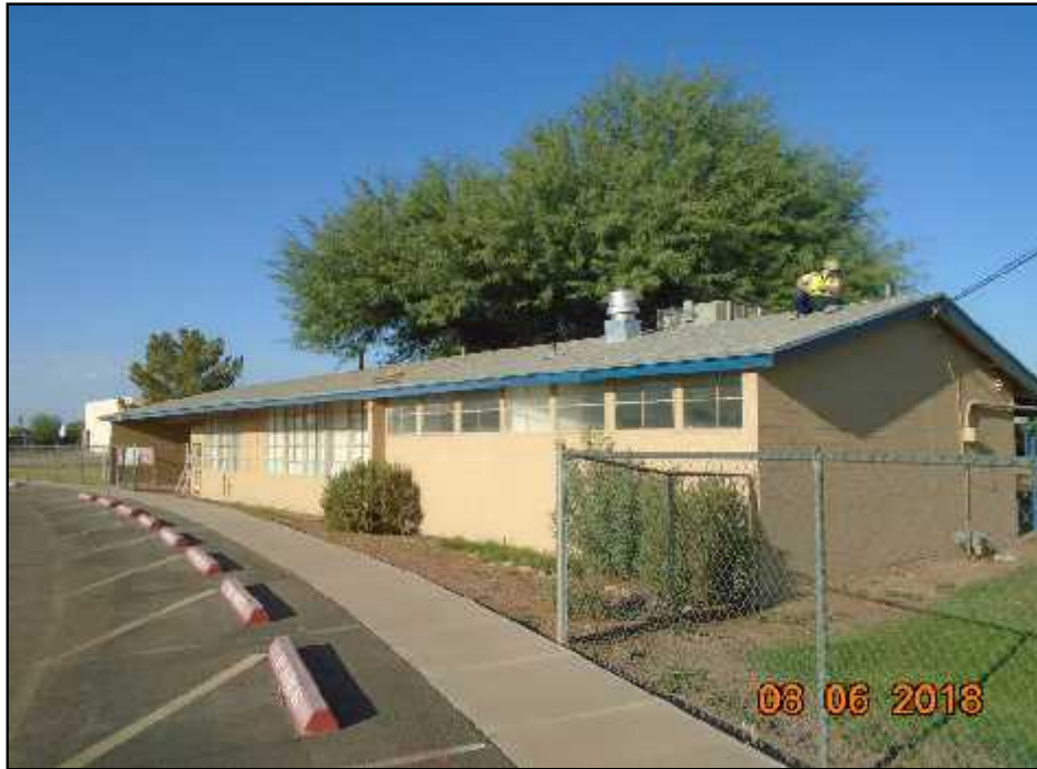
Picture 1 – East side exterior of Building 5 (RPA Building H).
