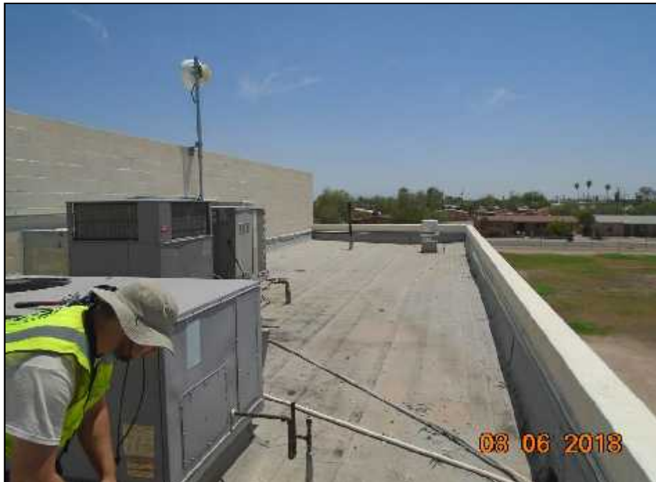
Picture 14 – Roof of Gymnasium (RPA Building G).
