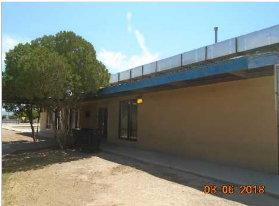
Picture 10 – North side exterior of Building 14 (RPA Building F).
