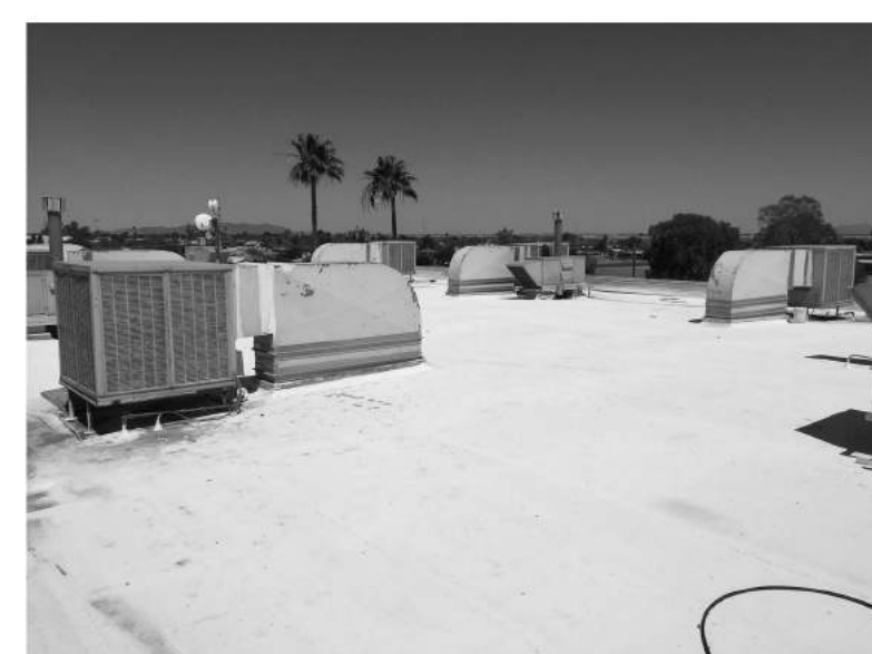
UPPER ROOF LEVEL
