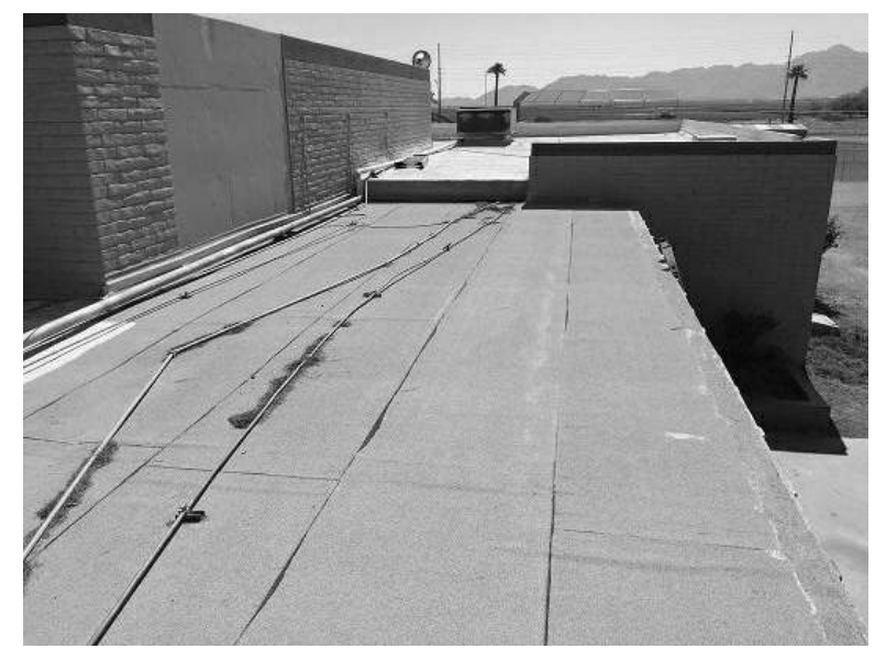
WALKWAY ROOF AT CAFETERIA
