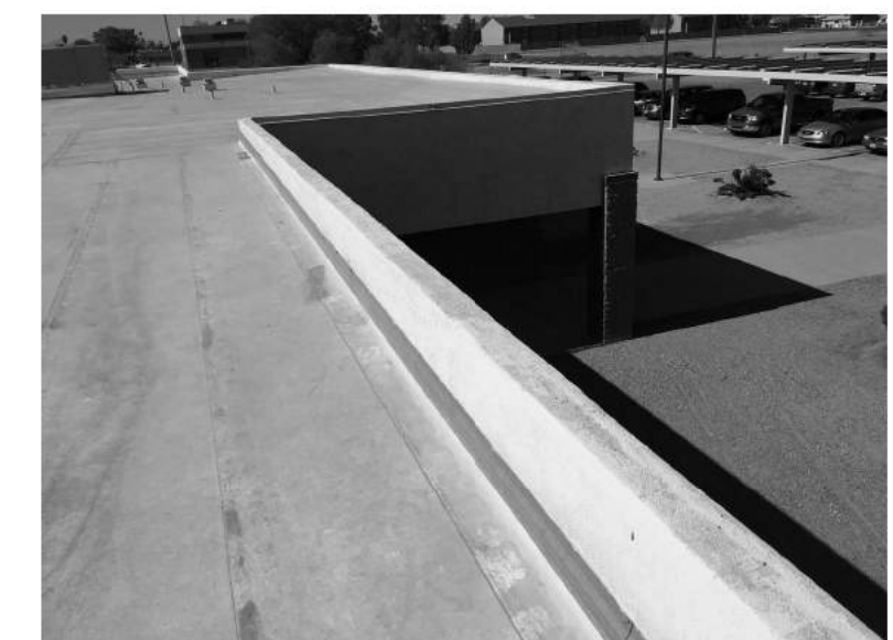
EXISTING LOWER ROOF PARAPET
