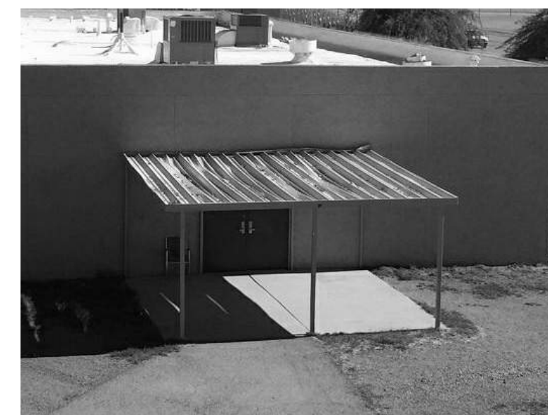
LOCKER BUILDING CANOPY
