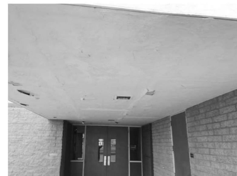
ENTRY SOFFIT, DOORS AND FRAMES
