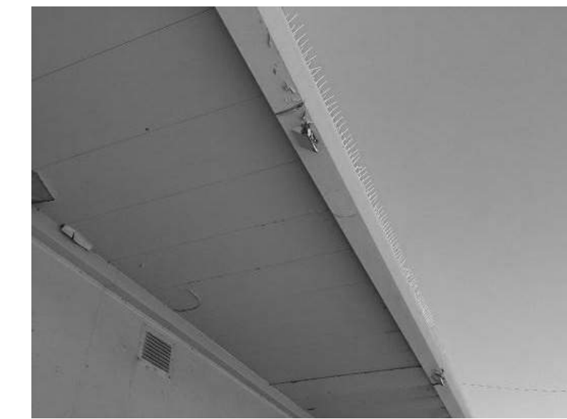
BAND BUILDING SOFFITS - REPAINT
