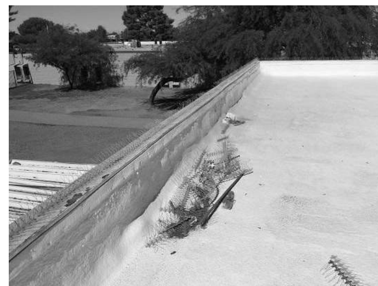
LOCKER BUILDING PARAPET
