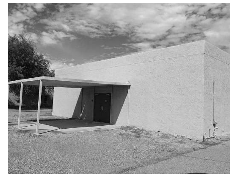
LOCKER BUILDING STUCCO WALLS
