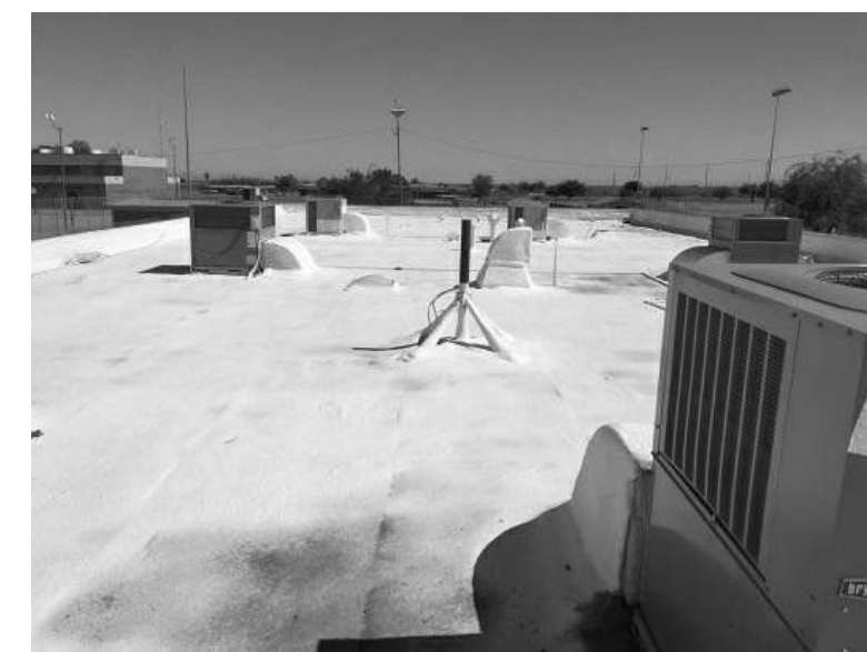
LOCKER BUILDING ROOF
