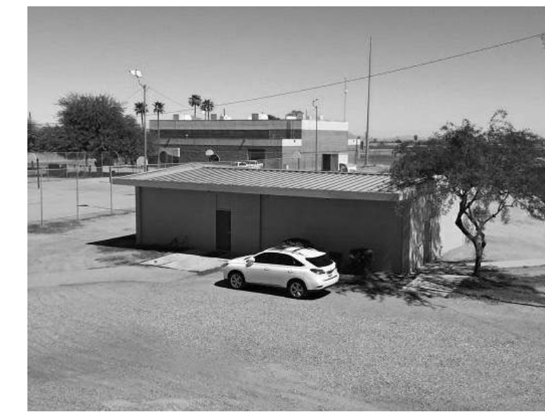
BAND BUILDING - REPAINT SOFFITS
